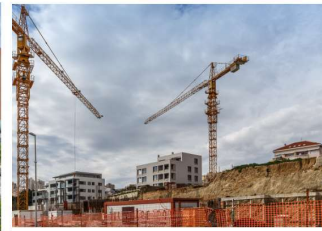
Construction Job Site
