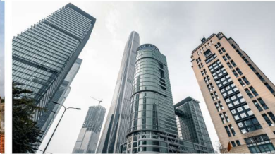
Office Building Job Site
