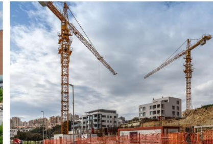
Construction Job Site
