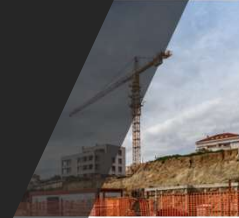
Construction Job Site
